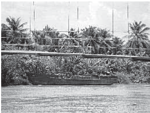
Suspension bridge used to get to House #1
